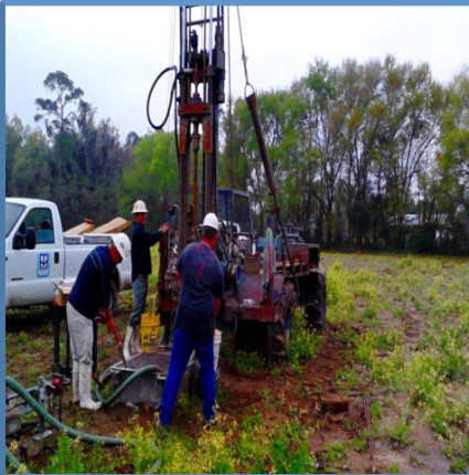
Geotechnical and Hydrogeological Boring
